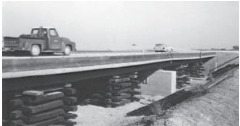
Cribbing placed below test bridges.
