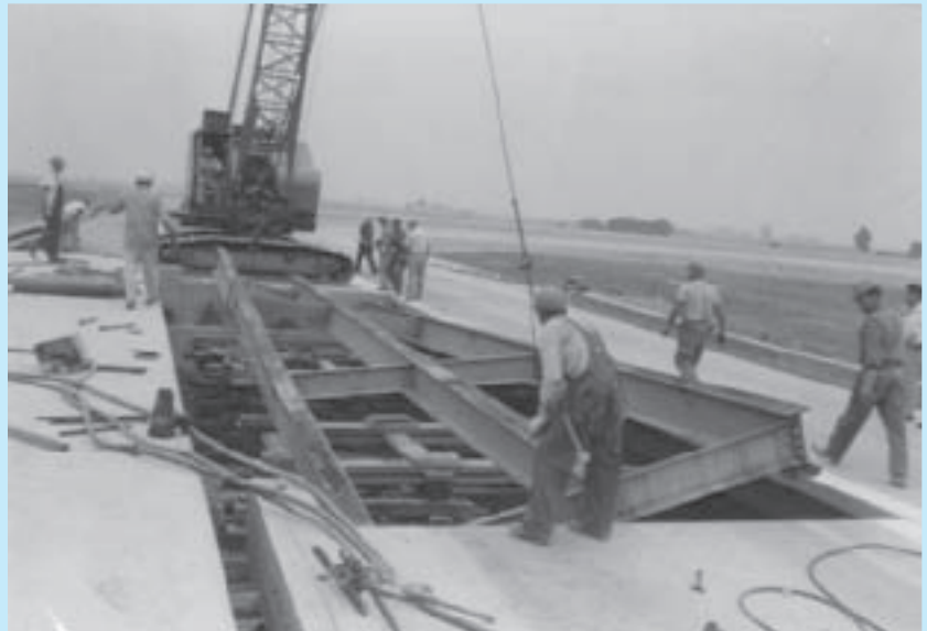
Removing damaged steel from test bridge.
