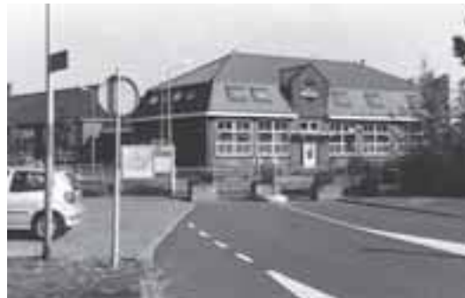
Disconnected neighborhood access road near Margriet primary school.
