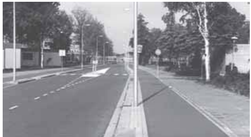
New cycle lanes and a pedestrian crossing at Steenen Kamer school.
