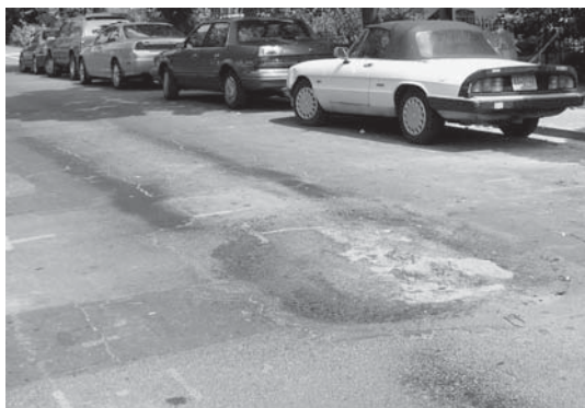
Pavement patches in Washington, D.C.
