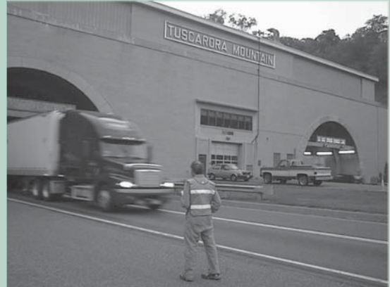
Fleet average and light- and heavy-duty vehicle emissions data from tunnel studies (above, Tuscarora Mountain Tunnel, Pennsylvania Turnpike) were used to determine and validate MOBILE 6 model performance.
