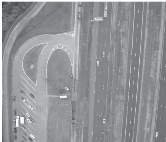
Aerial view of major highway from mini-UAV.
