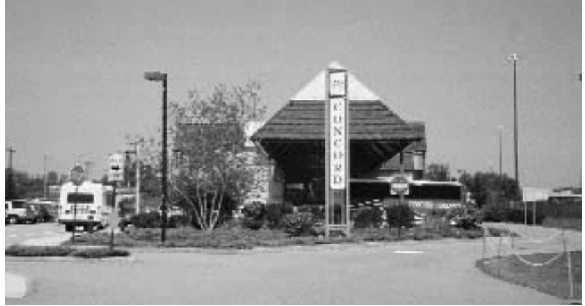
New Hampshire Department of Transportation built the Concord station, with a park-and-ride lot, local rural and small urban transit, intercity bus service, and frequent service to airports and to the Amtrak station in Boston, Massachusetts.
