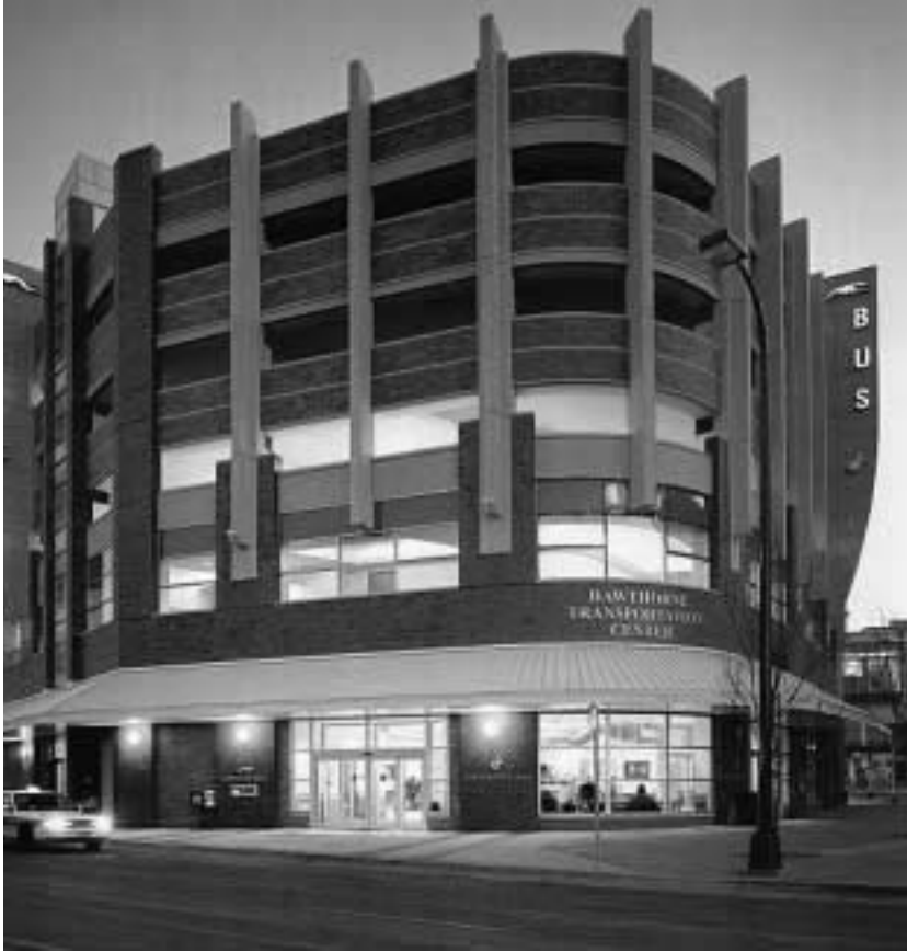
Hawthorne Transportation Center has revitalized the Minneapolis, Minnesota, downtown area, offering bus and transit connections to rural communities, public parking, and municipal offices.
