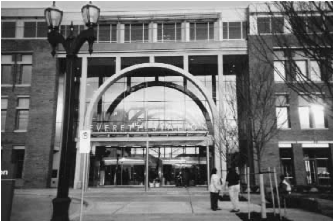
Everett Station in Washington State is an intermodal, educational, and employment services hub.
