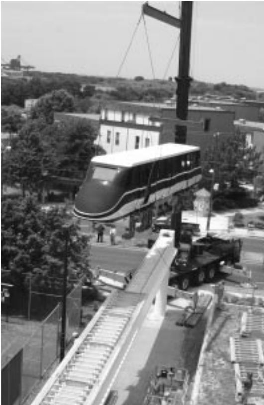
Maglev vehicle is maneuvered to position on guideway on campus of Old Dominion University, Norfolk, Virginia, but awaits funds for completion and operation.
