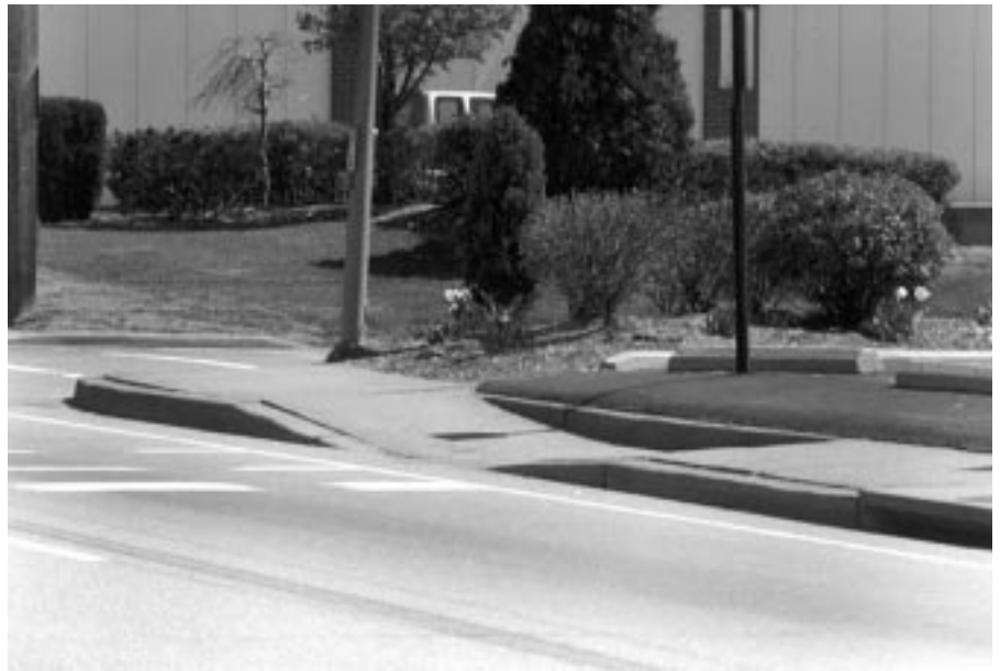
FIGURE 3 Sidewalk curb ramp.
