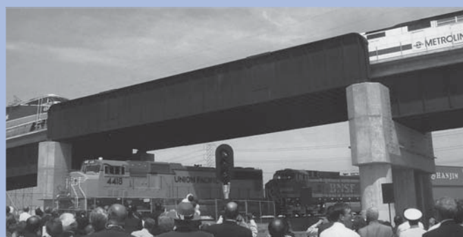
Redondo Junction flyover, shown during August 2001 dedication ceremony in Los Angeles, California, carries passenger trains over freight rail lines, surface streets, and the Los Angeles River on a bridge more than 800 yards long.
