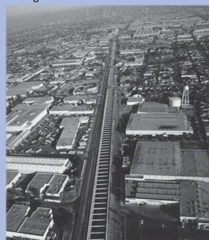
The Mid-Corridor Trench—the signature element of the Alameda Corridor—is 33 feet deep and 50 feet wide and stretches for 10 miles along Alameda Street between State Route 91 in Compton and 25th Street in Los Angeles.
