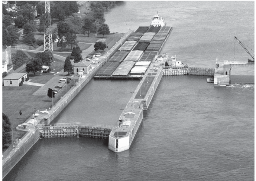
Tow approaching small lock, Upper Mississippi River. Small locks and higher average horsepower tows contribute to river's lower efficiency rating.
