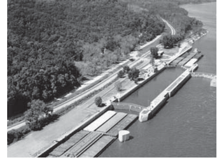
Tow cuts passing through Lock and Dam 22 on Upper Mississippi River.
