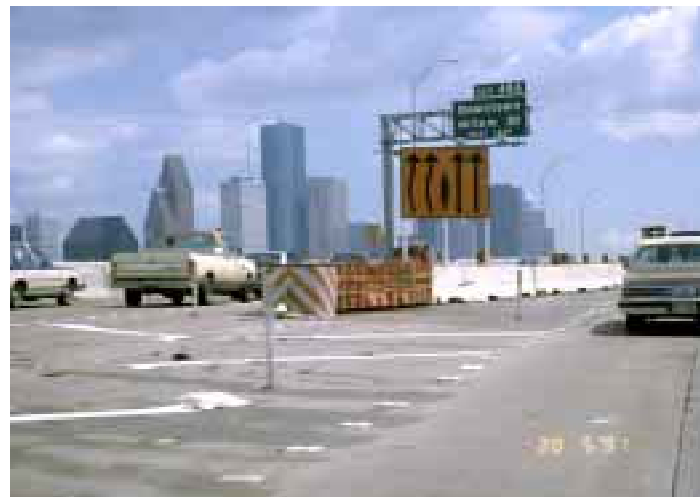
Figure 22 Example of Additional Signing and Delineation Needed for a Traffic Split on a High-Volume Roadway
