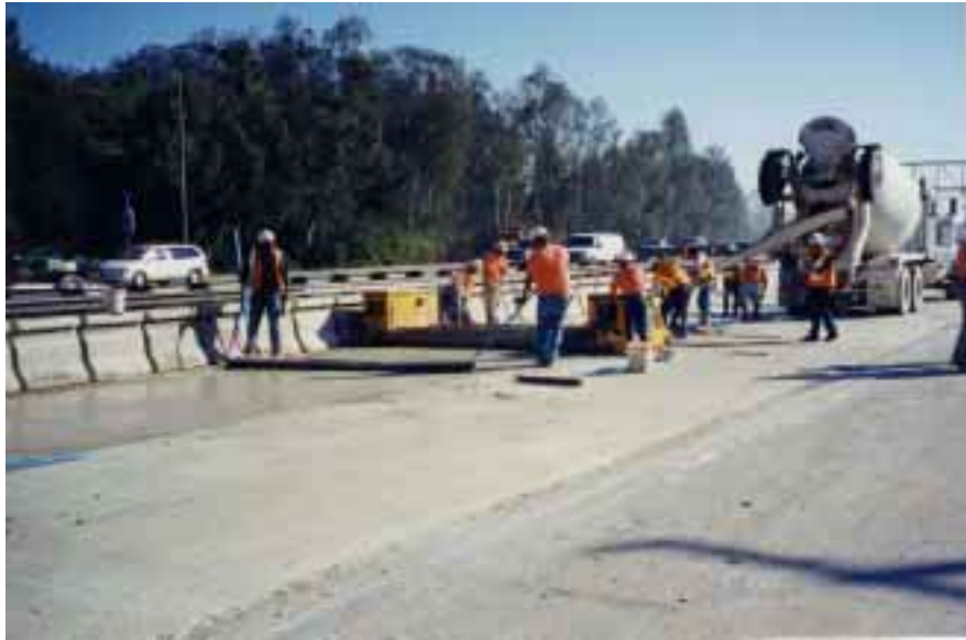
Figure B.5 Safe work zone area, I-10 Pomona, California
