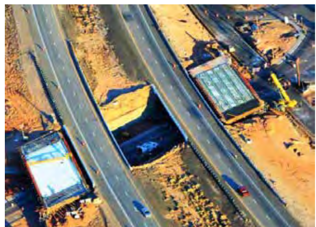
FIGURE 32 Mesquite Overpass project prior to bridge slide (Searcy and Kolkman 2012).
