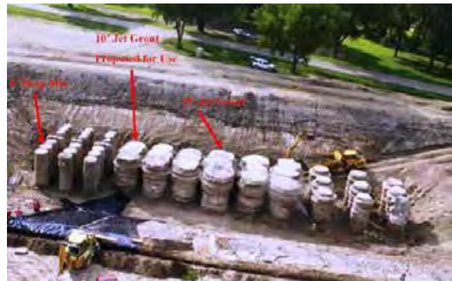
FIGURE 19 Jet-grouted samples prior to destructive testing (Note the size of the samples compared with the size of the equipment in the picture) (Hoffman et al. 2009).
