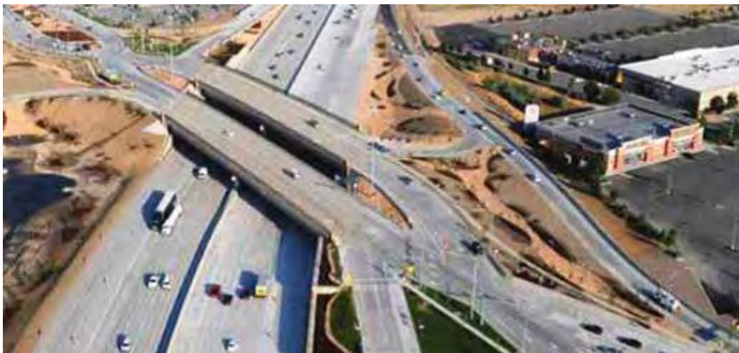
FIGURE 30 Completed diverging diamond interchange at Pioneer Crossing (Haines 2011).
