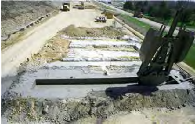
FIGURE 18 Jet grouting in progress (Trevicos 2010).
