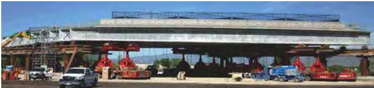
FIGURE 29 Pioneer Crossing Bridge being put in place by SPMTs (Haines 2011).
