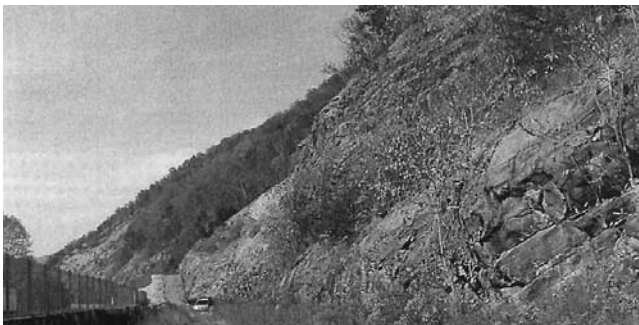
Figure 5-35. Rock slope at Pigeon Gorge, I-40 in North Carolina.
