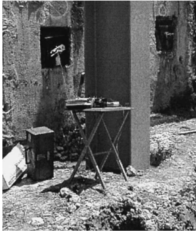
Figure 5-19. Electrical measurements being made at O Street wall, Washington, D.C.
