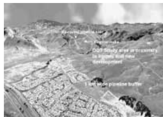
FIGURE 6 PG&E pipeline showing encroachment of neighborhoods inside the 1-km buffer.
