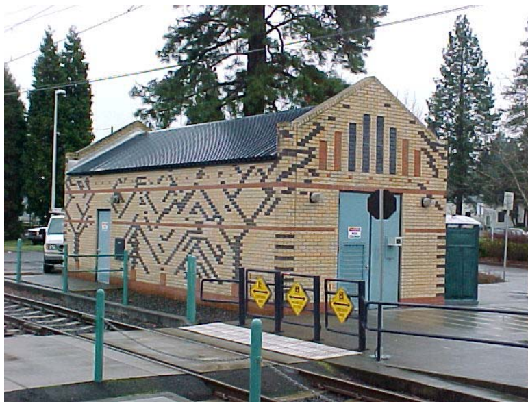
FIGURE 2 TriMet Westside LRT Expansion Millikan Substation, 1998.
