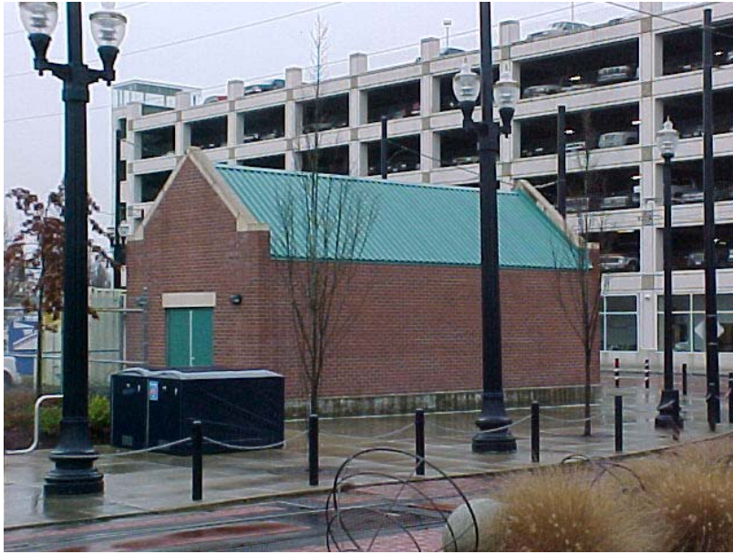
FIGURE 5 TriMet Hillsboro LRT Extension Government Center Substation, 1998.
