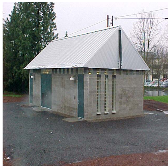
FIGURE 8 TriMet Interstate MAX LRT Failing Street Substation, 2003.
