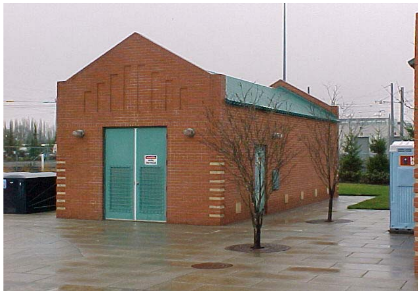
FIGURE 4 TriMet Westside LRT Expansion 170th Street Substation, 1998.
