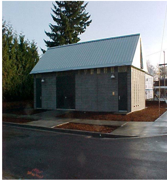
FIGURE 7 TriMet Interstate MAX LRT Killingsworth Station Substation, 2003.
