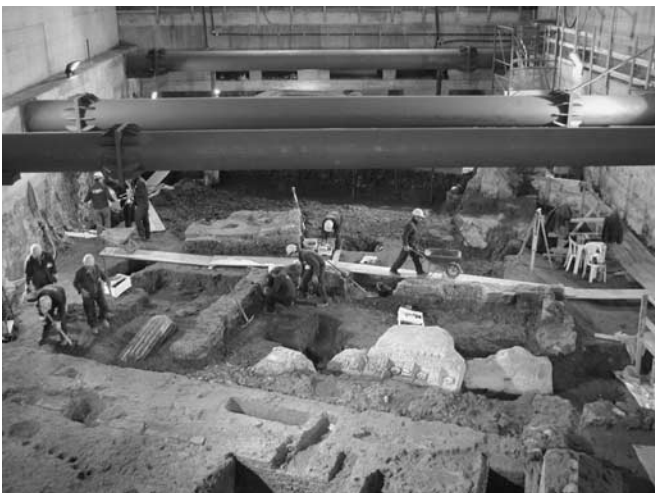
Figure 7 Duomo excavation site.
