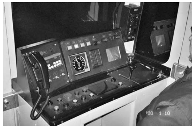
Figure 9 Milan's train operator console.
