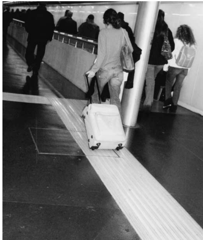
Figure 12 Guideways for the visually impaired at a station in Naples.
