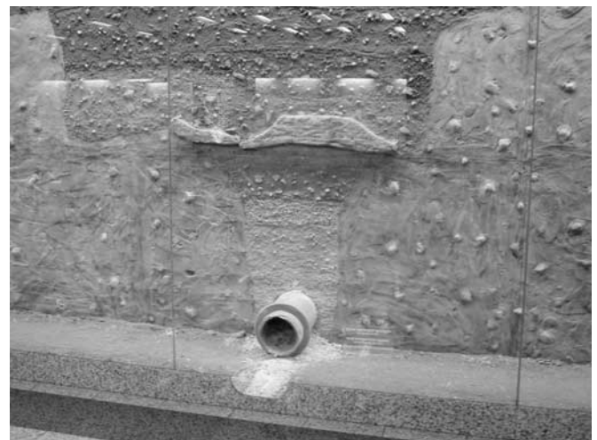
Figure 15 Terracotta pipes from the Pisistratid aqueduct.
