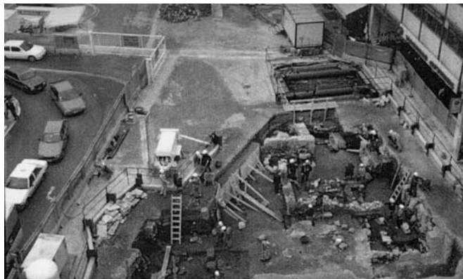
Figure 6 An excavation site in Athens.
