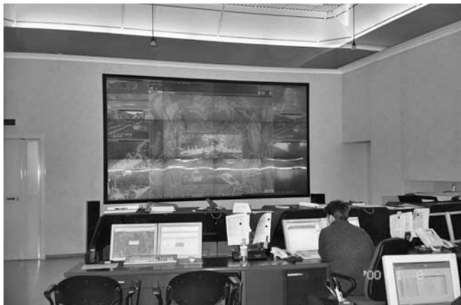
Figure 8 ITS Traffic Control Center managed by STA in Rome, Italy.
