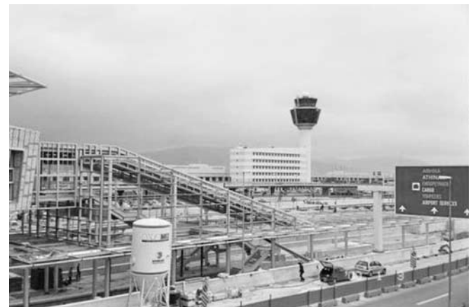
Figure 13 The intermodal airport station under construction.
