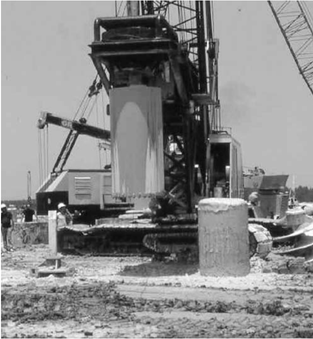
FIGURE 48 Intact rock core removed using crane-mounted rotary drill and core barrel.
