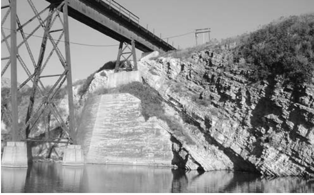
FIGURE 4 Bridge site with surface exposures of foundation rock.
