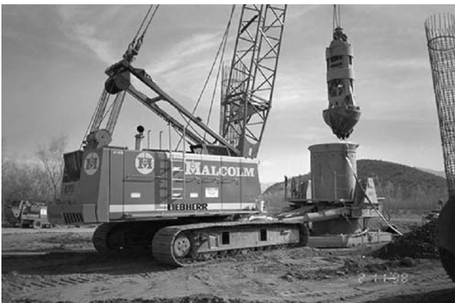
FIGURE 49 Casing oscillator and hammergrab tool.
