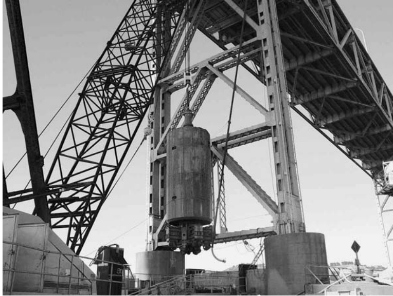
FIGURE 57 Shrouded bottom hole assembly lifted for placement through the top unit (Byles 2004).
