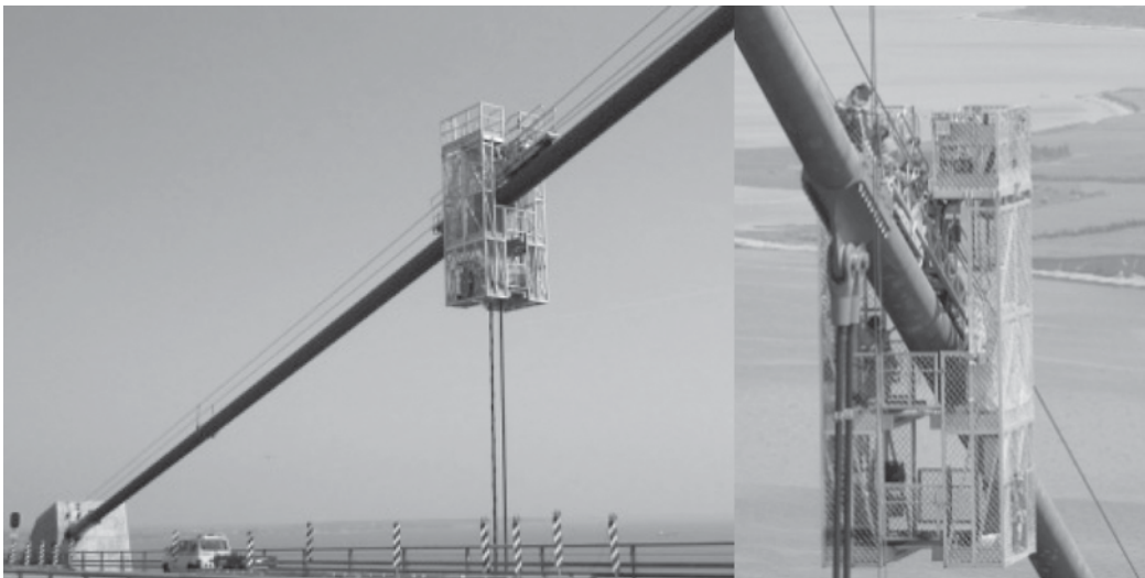
FIGURE 57 Carrier for inspection of main cable of suspension bridge in Denmark.
