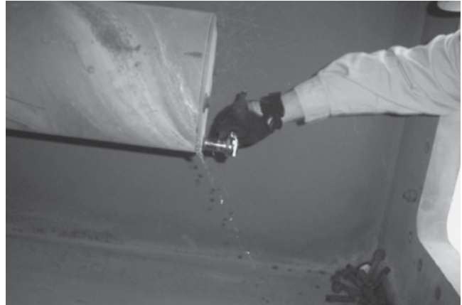
FIGURE 34 Water exiting the end cap of one anchorage (Telang et al. 2004).
