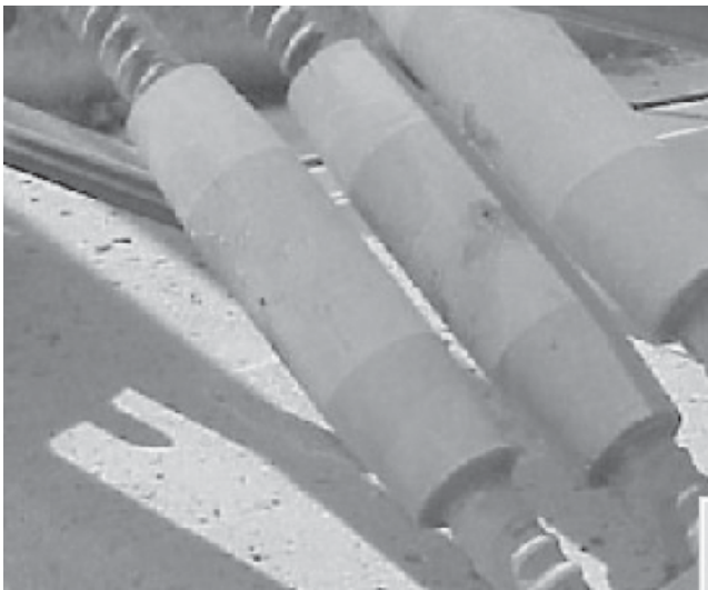
FIGURE 7 Typical bar couplers in stay cables.
