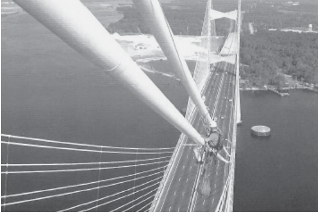
FIGURE 56 Rolling device for inspection of the stay cables on the Dame Point Bridge (“B&N Creates Custom Device . . .” 2005).
