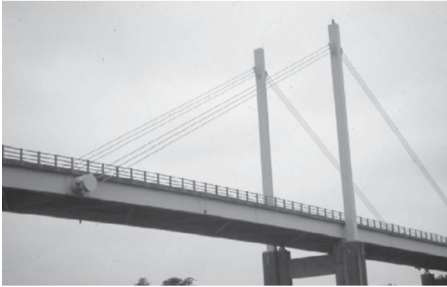
FIGURE 2 Sitka Harbor Bridge in Alaska, the oldest cable-stayed bridge in the United States (Frank and Breen 2004).
