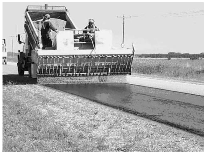
FIGURE 49 Aggregate applied with self-propelled spreader.
