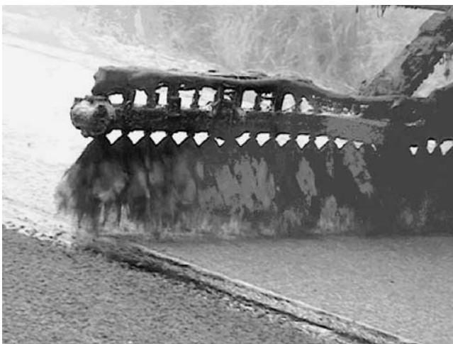
FIGURE 46 Spray bar applying bituminous binder.
