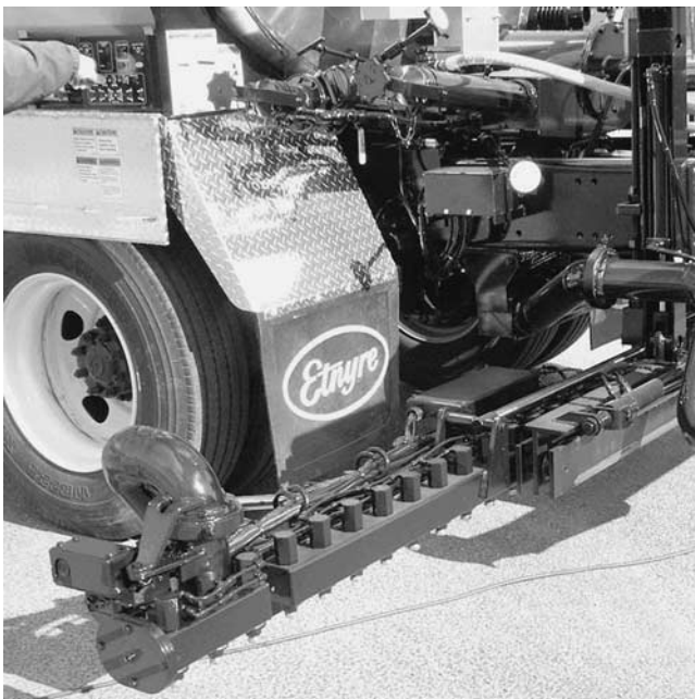
FIGURE 30 Distributor spray bar.
