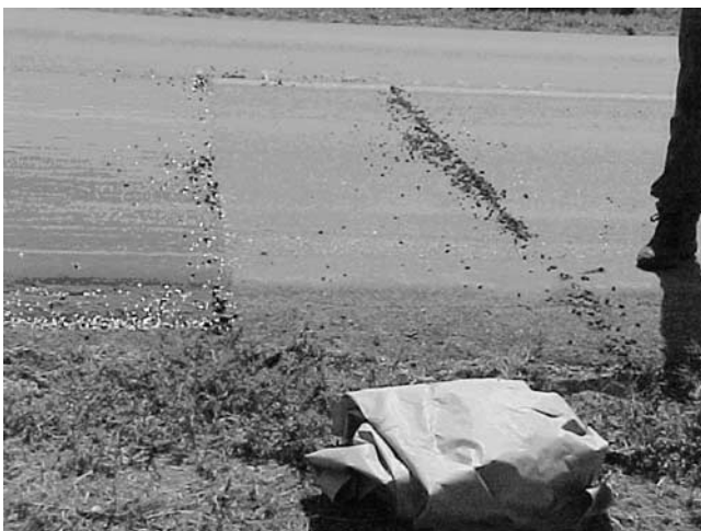
FIGURE 48 Paper used to ensure seamless transverse joint.
