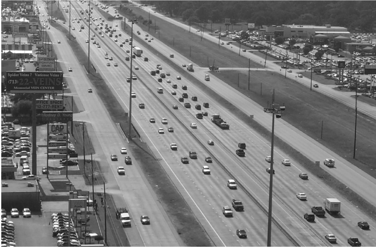
FIGURE 46 Reversible segment of the Katy Freeway, Houston, Tex. ["High Occupancy Vehicle (HOV) Interactive 1.0" 1996].
