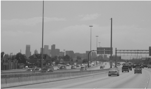
FIGURE 8 Reversible freeway segment with narrow cross section, Denver, Colo.
