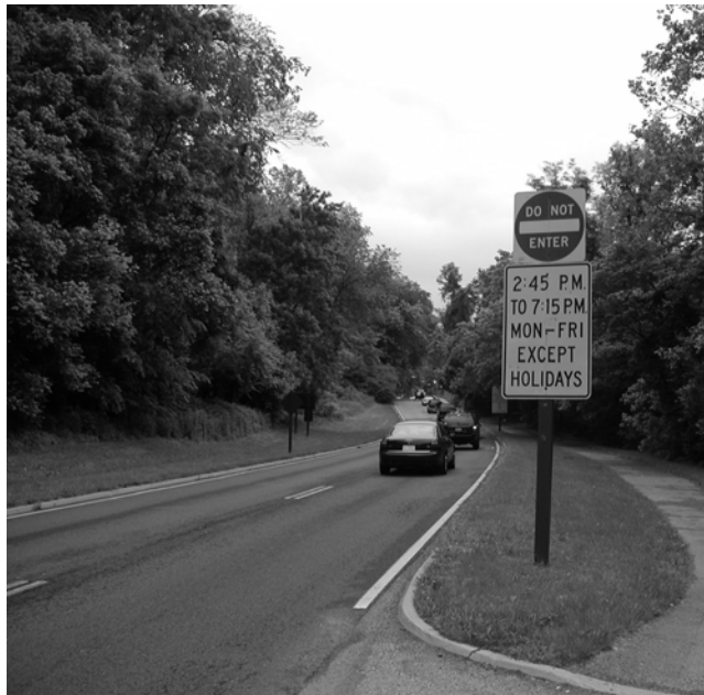
FIGURE 33 Canal Road—reversible lane segment, Washington, D.C.
