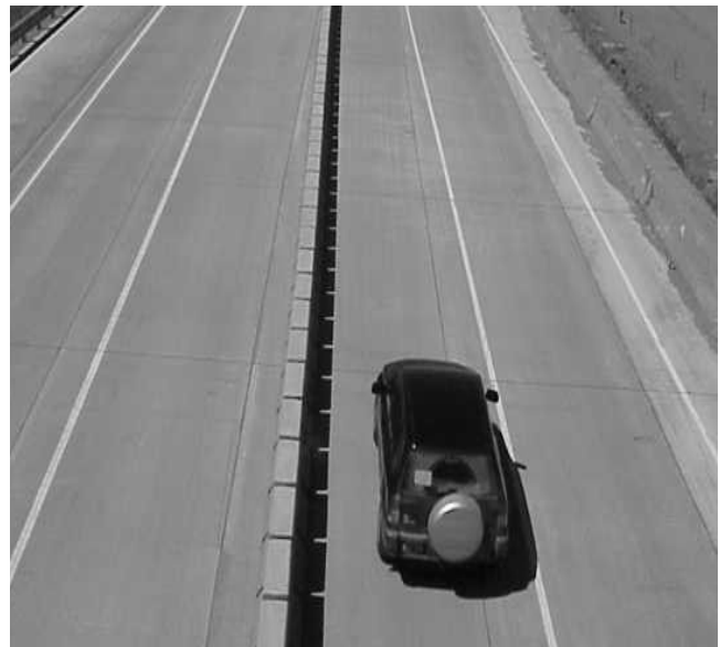
FIGURE 52 Overhead view of the use of shoulders as outer reversible lanes, Genesee County, Mich. (Courtesy: Armando Lopez, Michigan DOT).
