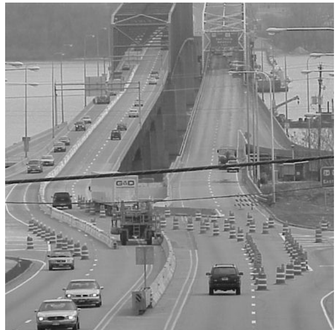
FIGURE 50 West entrance of the McClugage Bridge construction zone reversible segment, Peoria, Ill. ( Source : "Fact Sheet 5—Innovation During Bridge Rehabilitation Improves Mobility" 2003).
