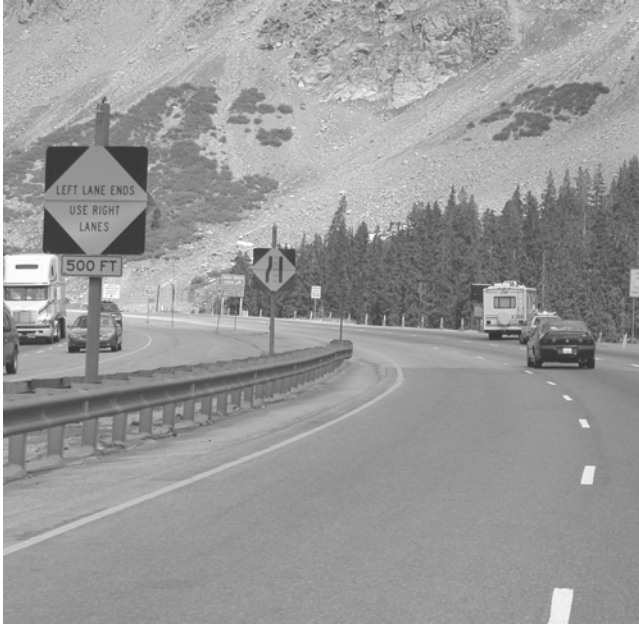
FIGURE 55 Eisenhower Tunnel flip-up signs (nonreverse flow operation), Summit County, Colo.
