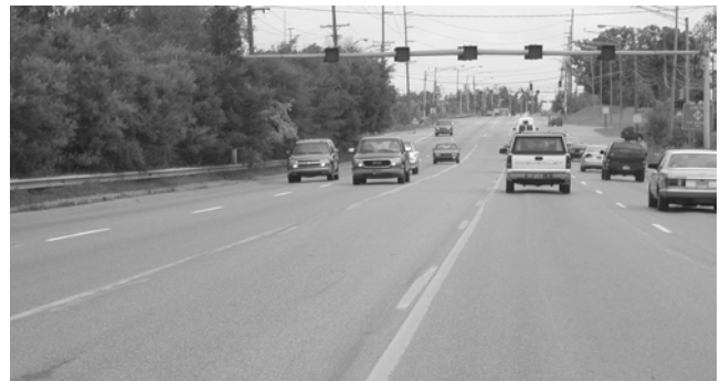
FIGURE 22 Deactivated lane-use signals and nonreversible pavement markings, Opdyke Road, Pontiac, Mich.
