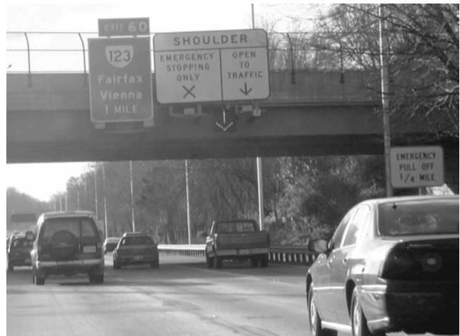
FIGURE 56 I-66 shoulder lane-use control sign and signal, Fairfax County, Va.
