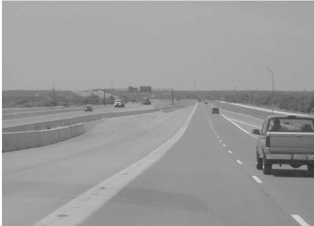
FIGURE 15 I-37 evacuation contraflow entry point, Corpus Christi, Tex. (Courtesy: Garry Ford, Texas Transportation Institute, San Antonio).
