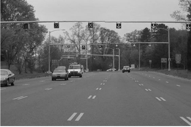
FIGURE 20 Overhead lane-use signals, Tyvola Road, Charlotte, N.C.
