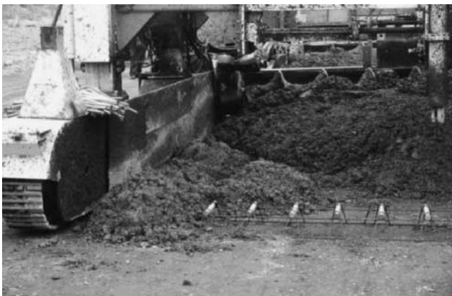
FIGURE 15 Concrete being placed over a dowel basket.
