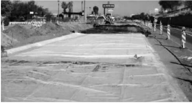
FIGURE 23 Polyethylene sheeting used as a curing method.
