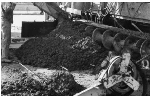
FIGURE 12 Use of a slipform paver.
