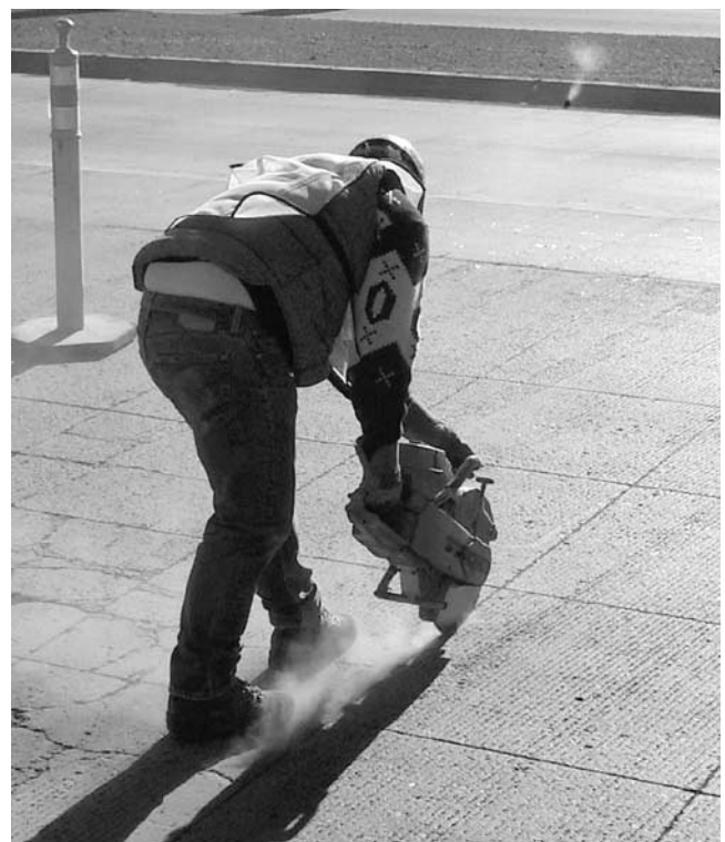
FIGURE 38 UTW repair step 1—Outline sawing.
