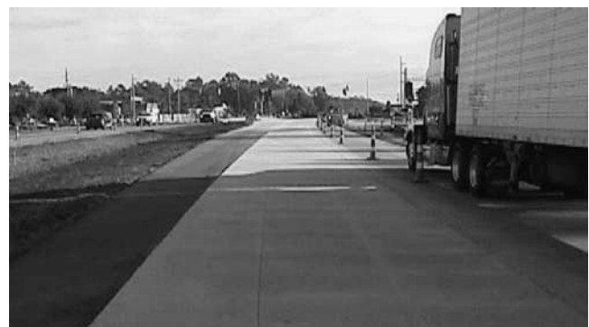
FIGURE 27 New shoulders meeting a new whitetopping elevation.
