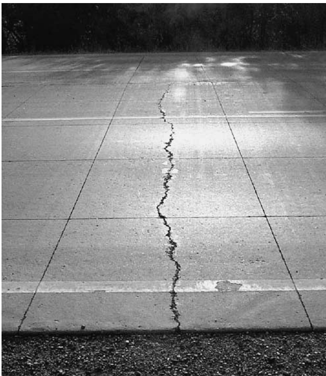
FIGURE 32 Typical midpanel crack on a TWT.
