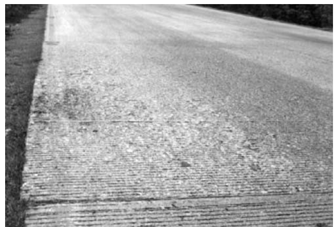
FIGURE 37 Typical surface wear.
