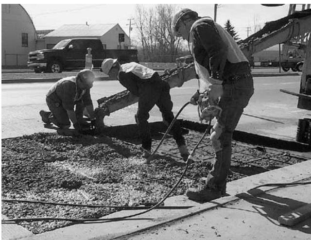
FIGURE 40 UTW repair step 3—Place new PCC.
