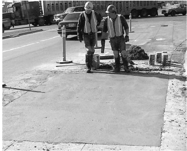
FIGURE 41 UTW repair step 4—Finish and cure PCC.
