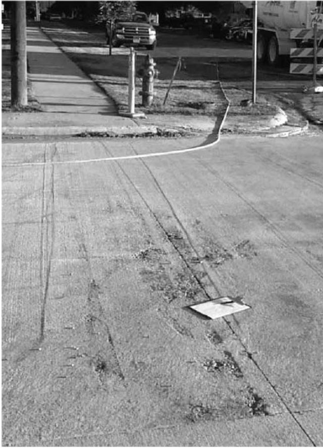
FIGURE 14 Poor consolidation.
