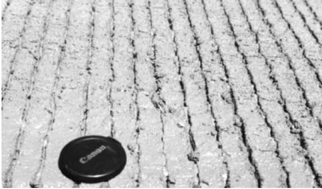
FIGURE 21 Tining comb texturization on freshly placed concrete.
