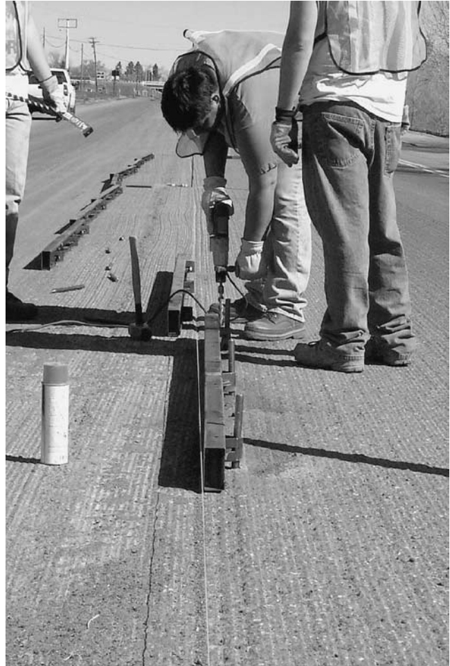
FIGURE 8 Use of fixed forms.
