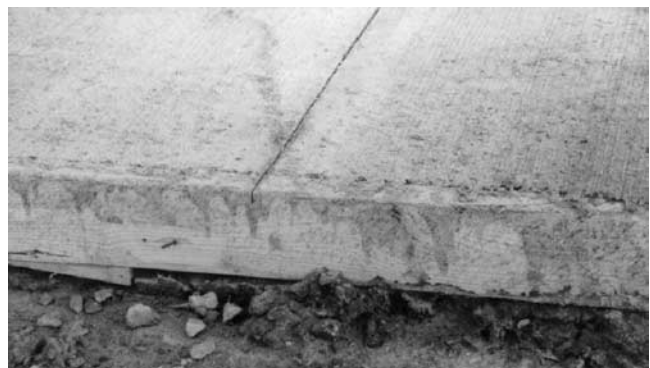
FIGURE 25 Sawcut depth using an early-age saw.
