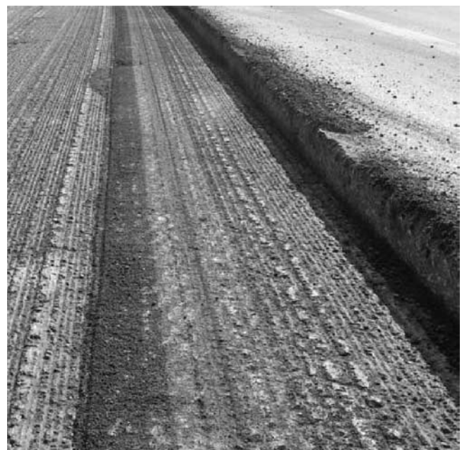
FIGURE 7 Milled HMA surface before overlay.
