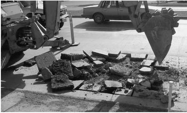
FIGURE 39 UTW repair step 2—Removing panels.
