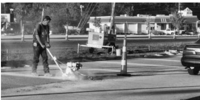
FIGURE 24 Sawcutting on a fast-tracked UWT.
