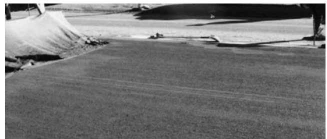
FIGURE 19 Application of texture with a burlap drag.
