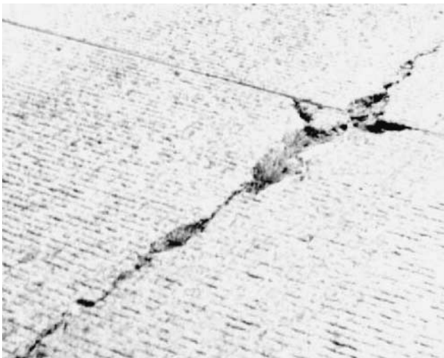
FIGURE 36 Severely spalled crack.
