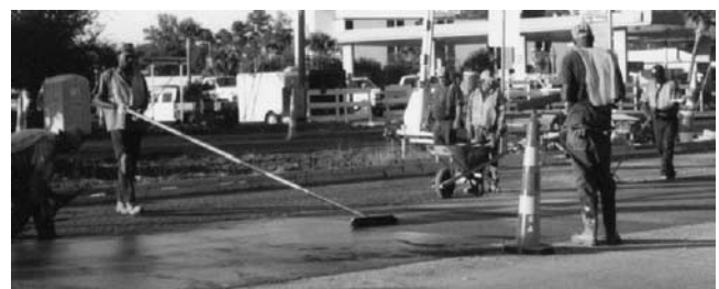
FIGURE 20 Application of texture with a coarse broom.
