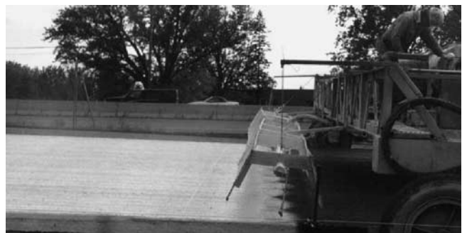
FIGURE 22 White-pigmented, liquid membrane curing compound.
