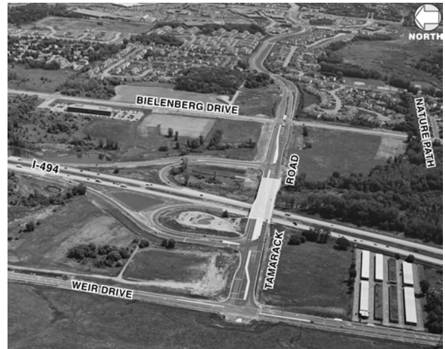
FIGURE 28 Tamarack Road/I-494 interchange after the project.
