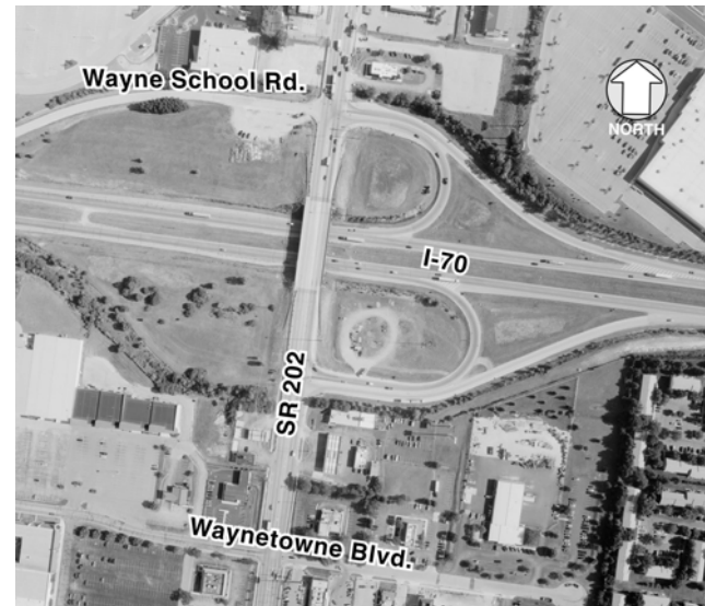
FIGURE 30 SR-202/I-70 interchange before the interchange modification study (Courtesy: Ohio DOT).
