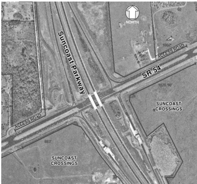
FIGURE 21 SR-54/Suncoast Parkway interchange after the project (Courtesy: Florida DOT).
