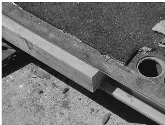
Figure 3.7.3.1.1-2 Shear key on Schuyler Heim decks.
