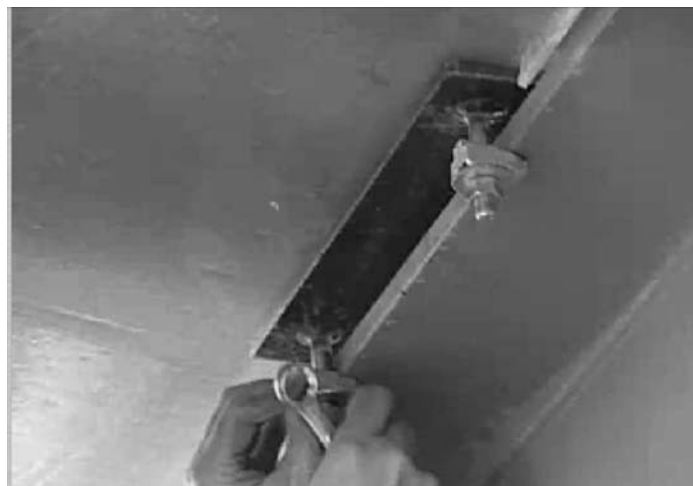
Figure 3.7.3.2.3-2 Girder clips for Jay Street Bridge.
