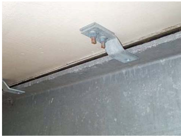
Figure 5.2.1.2-2 Clip type connection.
