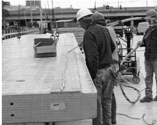
Figure 3.7.3.1.3-2 Application of adhesive on splice plates (Salem Avenue Bridge).
