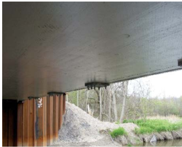
Figure 5.2.1.5-3 Underside of railing showing connection of railing to deck.
