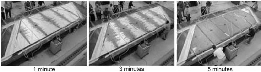
Figure 3.5.2-1 Vacuum infusion process on Tycor reinforced bridge deck.
