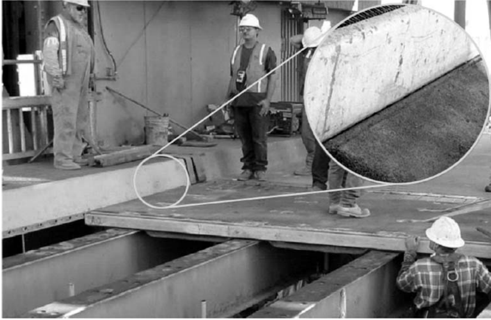
Figure 3.7.5.2-1 Curb and sidewalk adjacent but not connected to the FRP deck.
