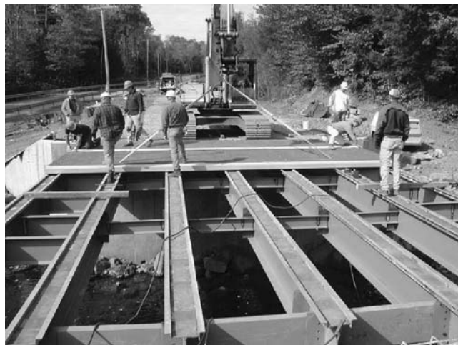
Figure 3.7.3.2.1-2 - Deck being laid down on steel girders; note the channel formed on the top flange for casting haunches.
