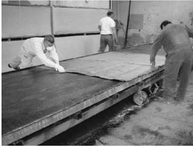
3.5.1-1 Hand lay-up operation: dry filament placement.
