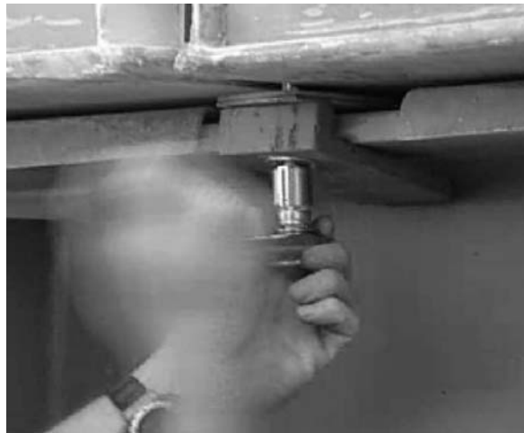
Figure 3.7.3.2.3-1 Anchor clips used on Jay Street Bridge.
