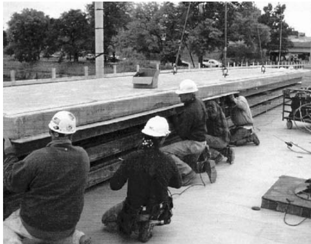
Figure 3.7.3.1.3-3 Mounting splice plates onto deck (Salem Avenue Bridge).
