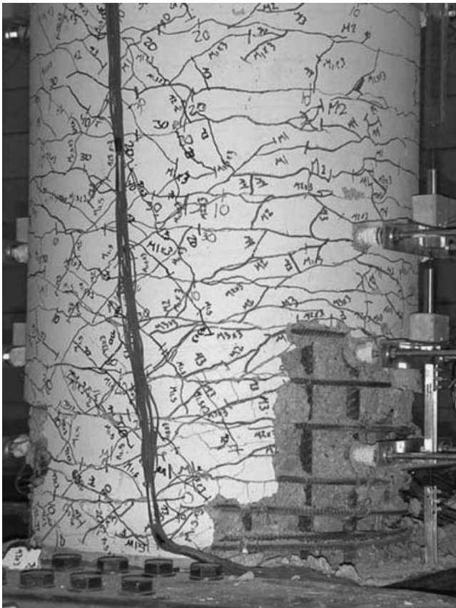
Figure 8. Partial view of column at the completion of seismic testing (SPC2, tension side of the column in the pull loading direction).
