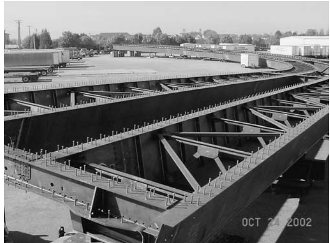
FIGURE 7 Special complete structure assembly (Washington State DOT).
