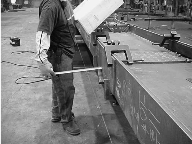
FIGURE 1 Measuring offset dimensions during shop assembly (Industrial Steel Construction, Inc.).
