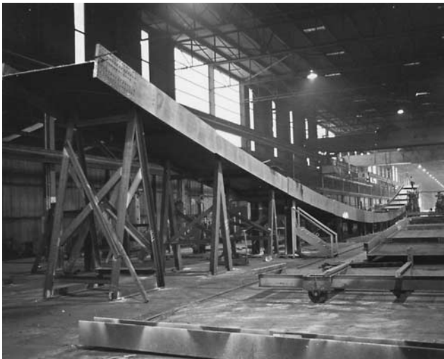
FIGURE 6 Progressive girder assembly.
