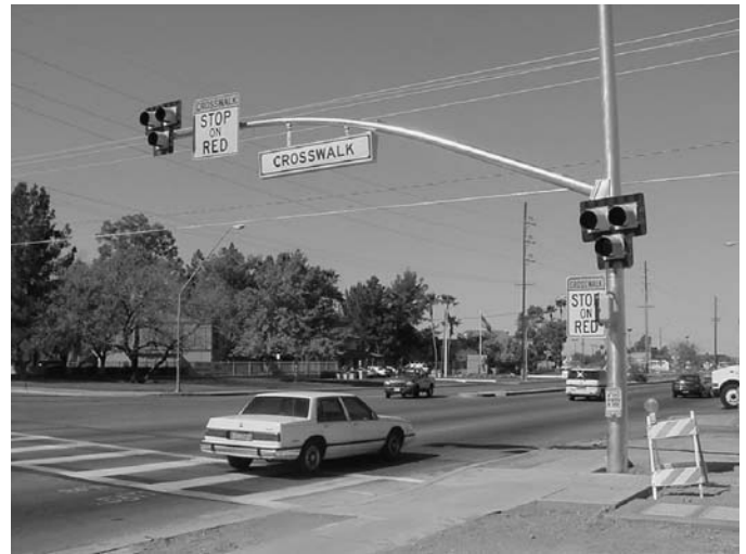
Figure 7. HAWK signal in Tucson, Arizona.
