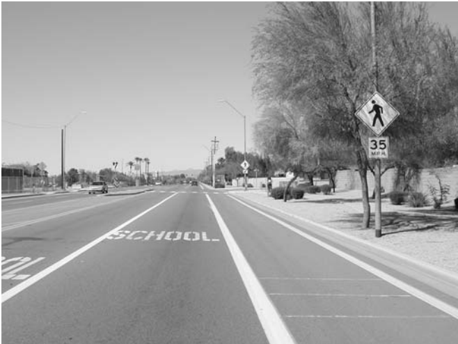
Advance Sign with Advisory Speed Plaque for School Crosswalk
