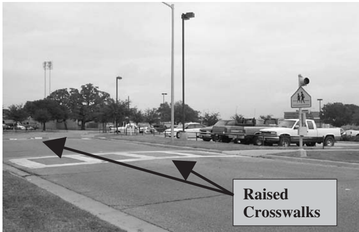
Raised Crosswalks with Supplemental Sign and Flashing Beacon
