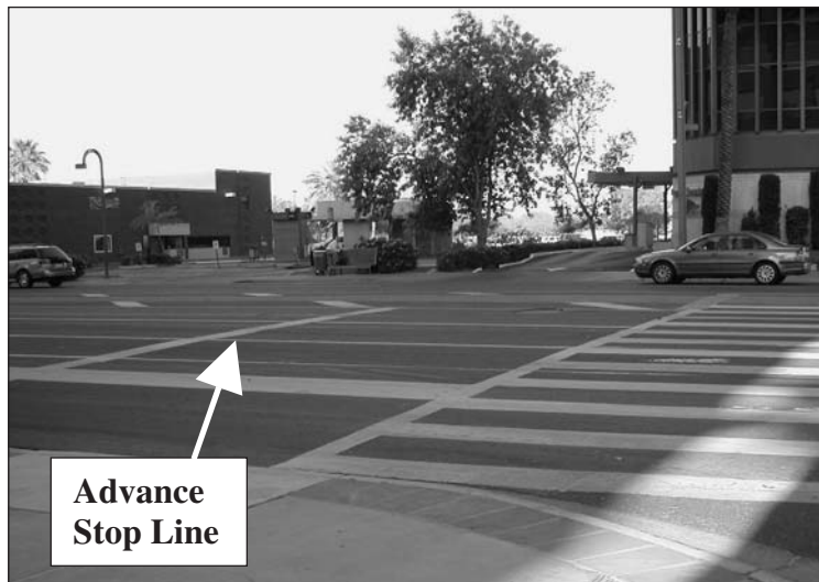
Advance Stop Line on Multi-lane Approach to Marked Crosswalk
