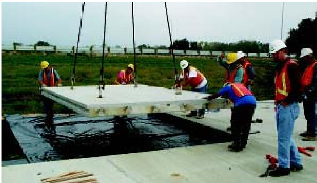
**FIGURE 5** Precast deck panel construction.
