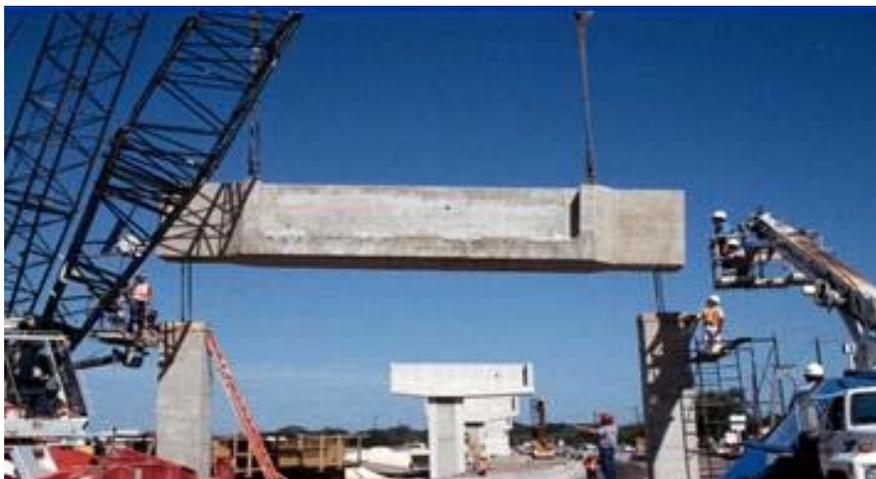
**FIGURE 8 Texas DOT precast, prestressed bridge construction.**
