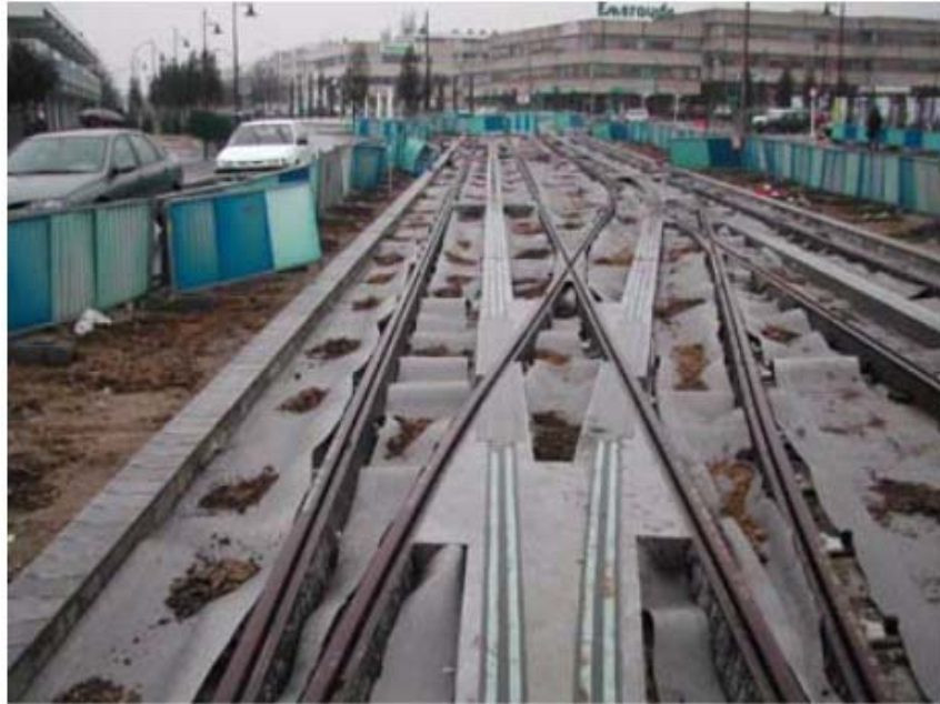
FIGURE 7 Crossing special trackwork.
