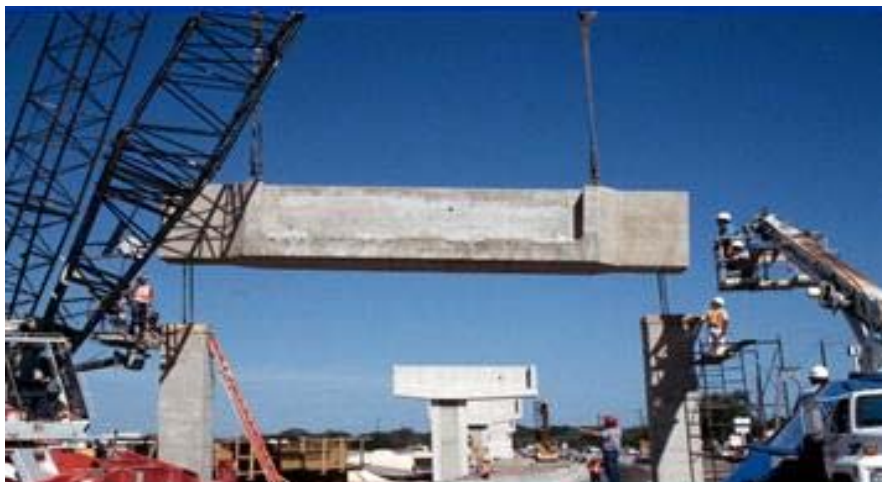
FIGURE 8 Texas DOT precast, prestressed bridge construction.
