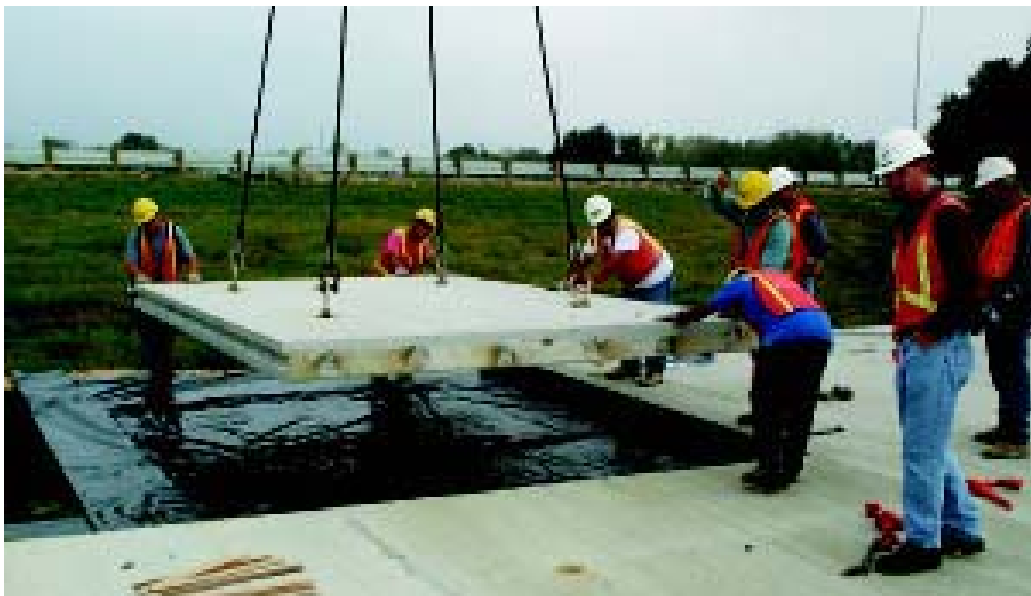
FIGURE 5 Precast deck panel construction.
