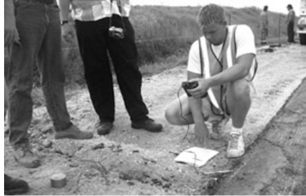
FIGURE 3 Nondestructive QC testing.
